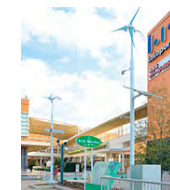
Wind turbines with attached solar panels LaLaport SHIN-MISATO
